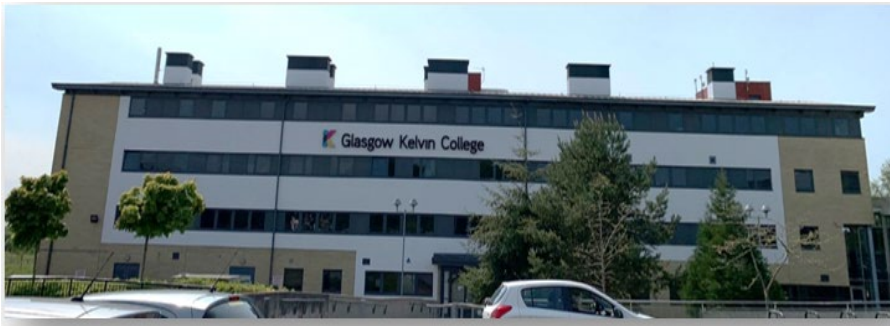
Repainted Exterior including Chimney Stacks
